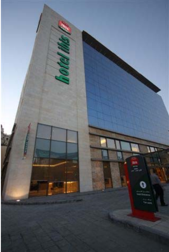
External view for the hotel
